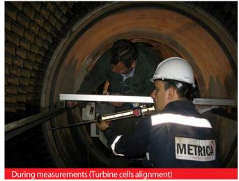
Gas-Turbine alignment: The main task was to define the geometric condition of the Gas-Turbine, make the necessary adjustment to achieve alignment and then re-measure to document and verify that the alignment was successful and within manufacturer tolerances. All processes were achieved successfully. The equipment that our team used was Easy Laser E 960B Turbine Alignment System.
