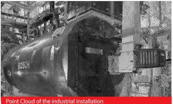
The first action was to place an adequate number of black and white targets all around the installation. Thes marks were well recognizable, and they had the size of an A4 paper. The installation was covered through 94 laser scanner setup positions with over 371 million points.
